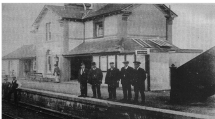
This picture shows the stationmaster's handsome residence, ticket office, luggage and waiting room and diner (now restaurant and lounge)
